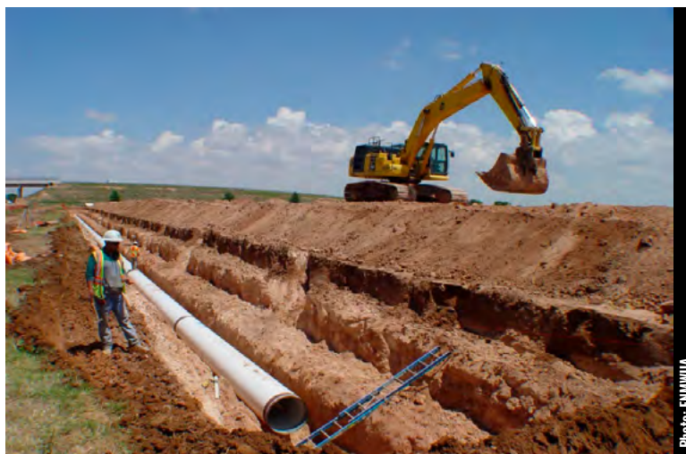
Progress is continuing on a pipeline to take water from Ute Lake to communities in eastern New México. Photo: ENMWUA
